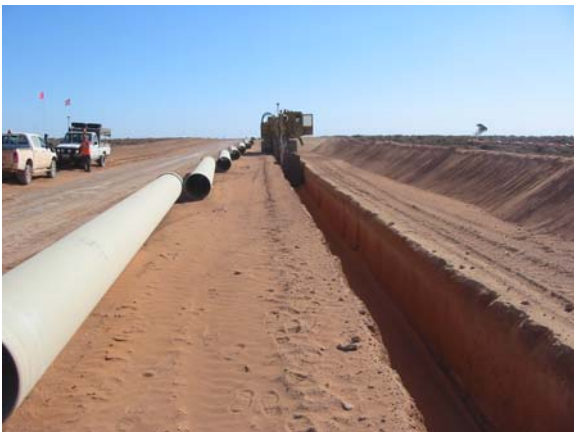
Figure 4: Pipe lengths “strung” along the alignment, ready for installation.
